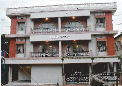
Completed: Rajalakshmi Lake Road, Manipal
